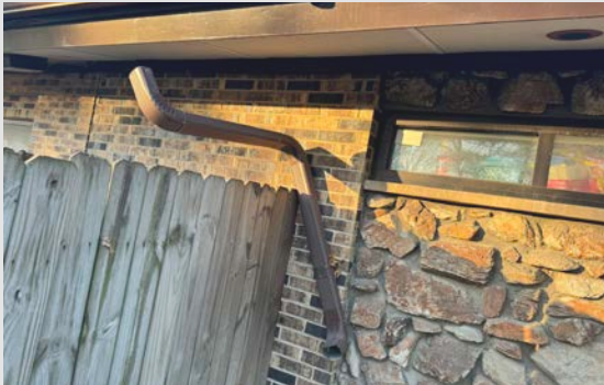
1 - Disconnected Downspout
