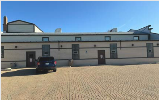
8 - Roofing - Single Ply Roofing
