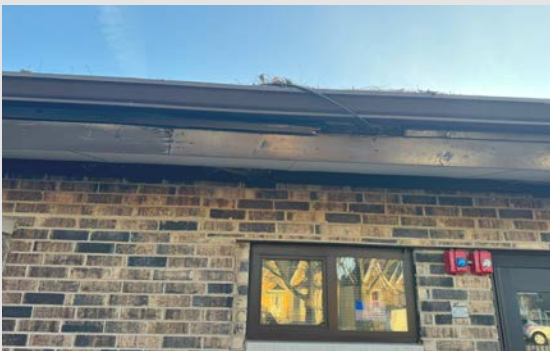
3 - Deteriorated Fascia
